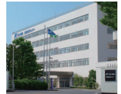
Facility Technology Center
